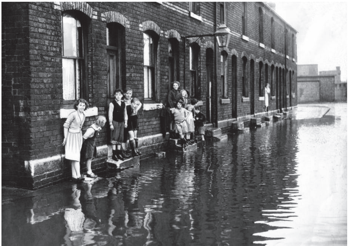
Figure 7 Floods at Surbiton Street, nr. Broughton Lane 20 th August 1954 (courtesy of Sheffield Newspapers)
