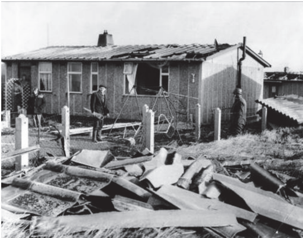
Figure 5 Damage to prefabs at Arbourthorne, February 1962 (courtesy of Sheffield Newspapers)
