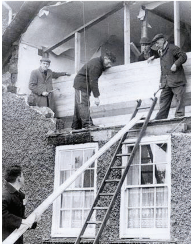
Figure 6 Damage to house on Heavygate Road, Walkley, February 1962 (courtesy of Sheffield Newspapers)
