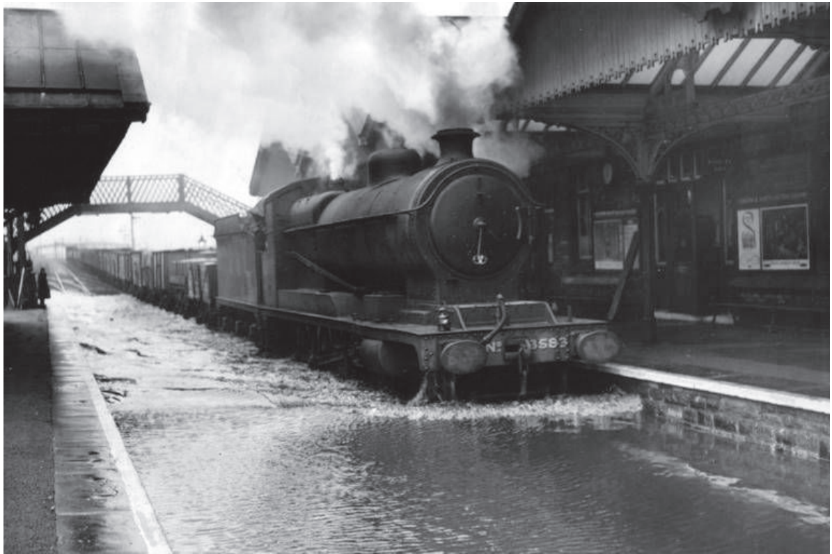
Figure 6 Floods at Beighton Station 3 rd February 1950 (courtesy of Sheffield Newspapers)
