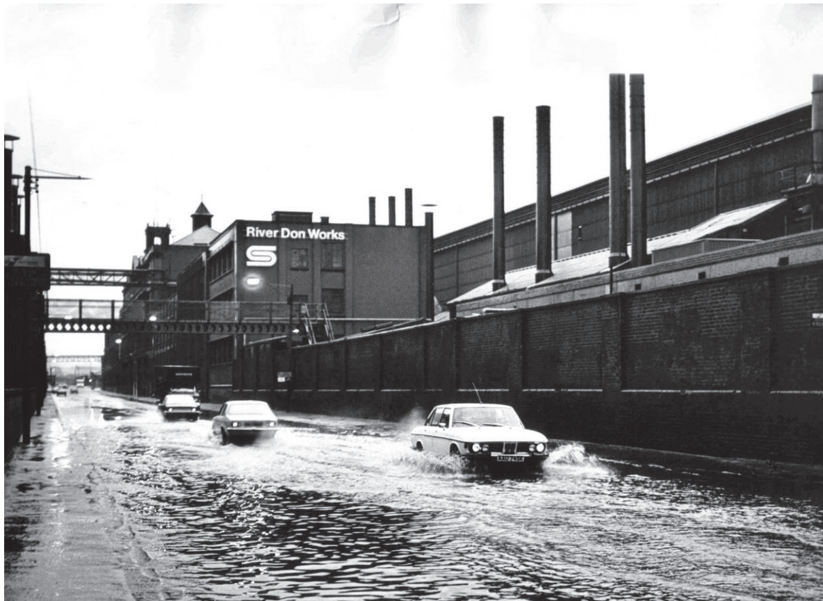
Figure 13 Floods alongside River Don Works 2 nd January 1978 (courtesy of Sheffield Newspapers)
